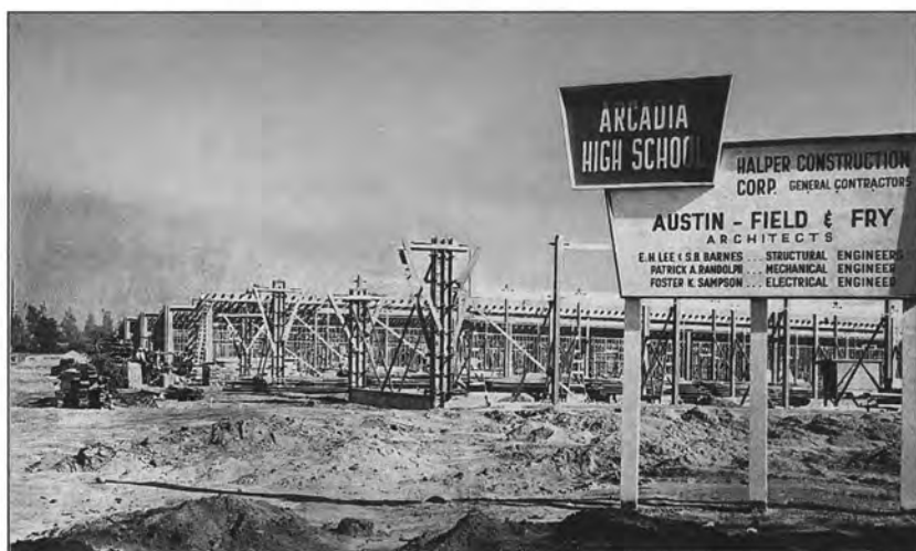
Arcadia High School under construction circa 1951. In June 1955, there were 342 seniors in the school's first graduating class.
