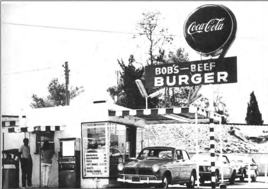
Bob's Beef Burger drive-through at 218 East Huntington Drive (southeast corner of East Huntington Drive and Second Avenue) circa 1969. It was demolished for a new retail center built in 1989.
